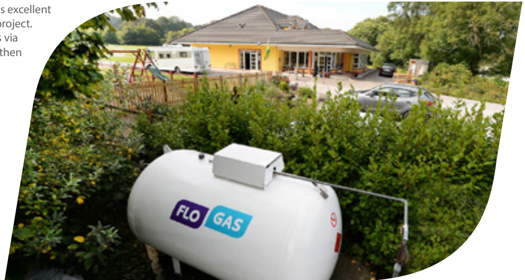
Flogas LPG tank
