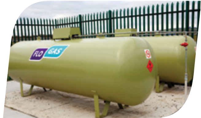
Flogas LPG tanks
